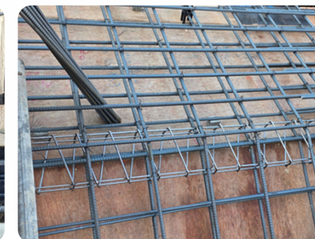
Tie three points with steel wire
