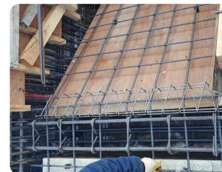
Place after installing internal horizontal bar
